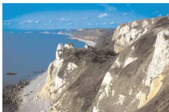
Historical and recent views of the Hooken landslide near Beer, East Devon. The slide occurred in 1789-90 and appears to have originated below sea-level. The drawing was made by Daniel Dunster in 1840, and the erosion of the front of the slide between then and the present day can be seen by comparing the two images.
