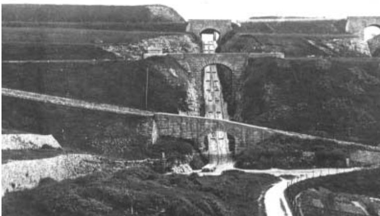
View of the incline plane at Portland used to transport stone to the harbour. Portland is a fine example of an industrial landscape resulting from limestone quarrying.
